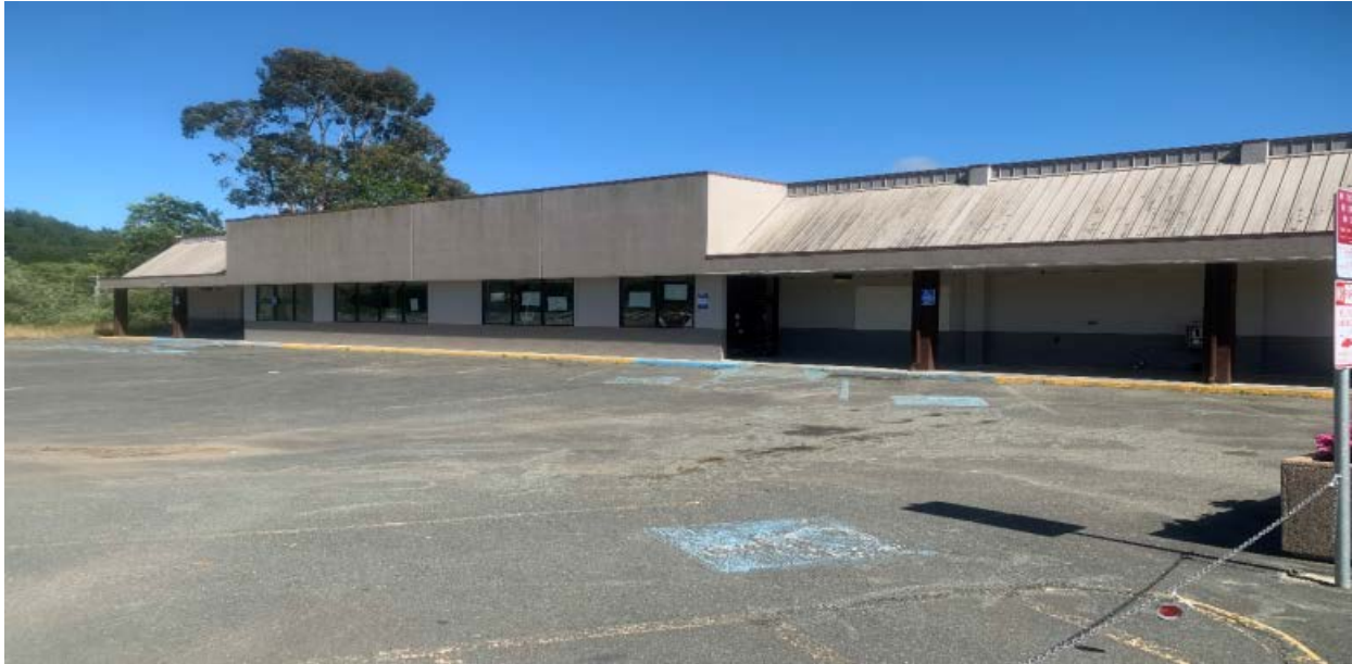
Smith River Fire Protection District, Future Station #1, 301 N. Fred Haight Drive, Smith River
