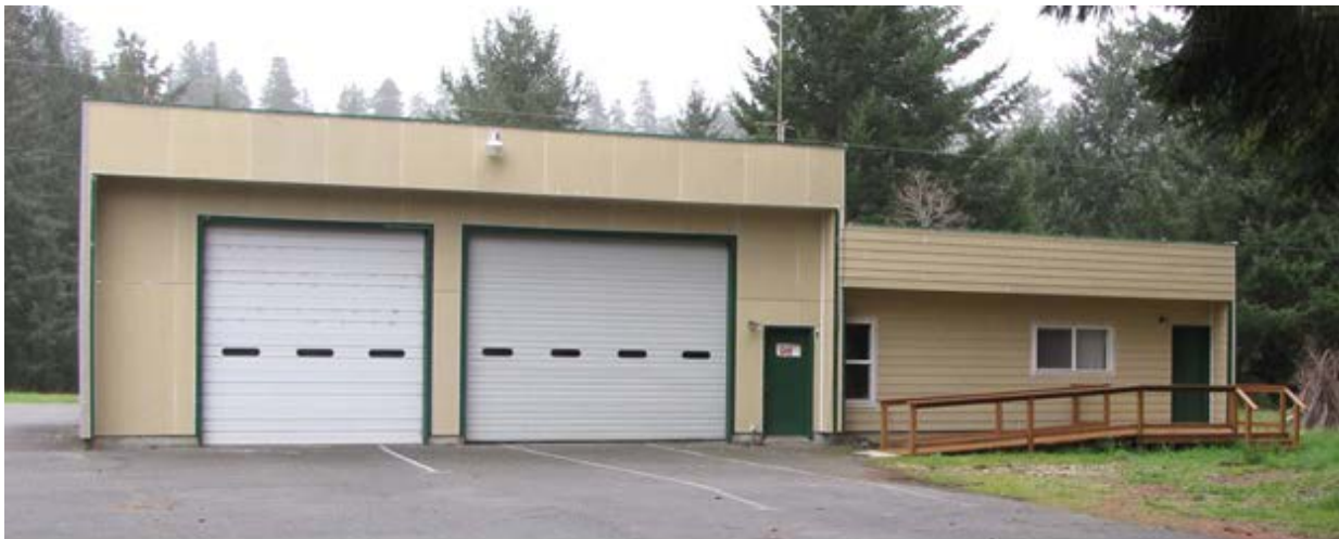
Smith River Fire Protection District, Station #2, 110 Dunklee Lane, Hiouchi, CA
